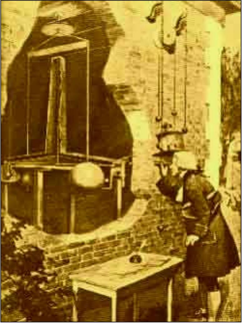
A cut away view of Cavendish's apparatus set in its closed chamber with observations being performed from outside.
